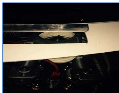
Figure 2b Fan & opening covers #3 & #4 cylinders only.
